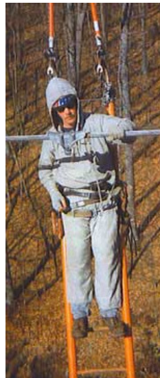
Bare-handed work on live transmission lines
