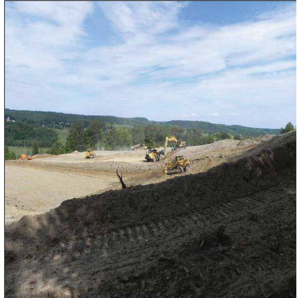
During well pad construction.
